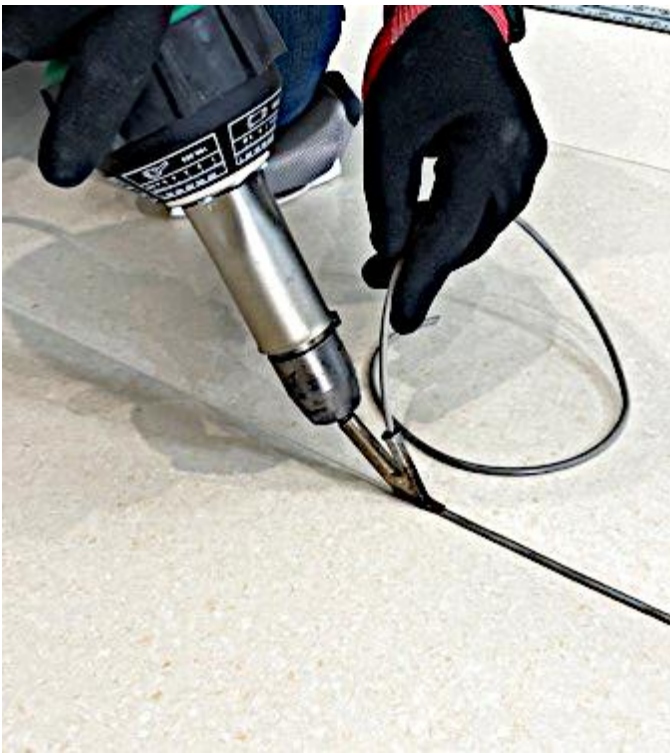
Figure 24 - Heat welding
