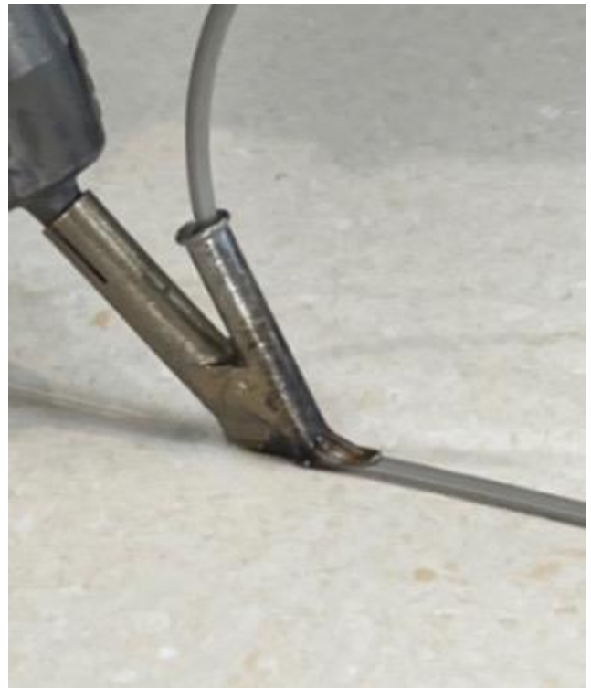
Figure 24 - Close up of heat welding
