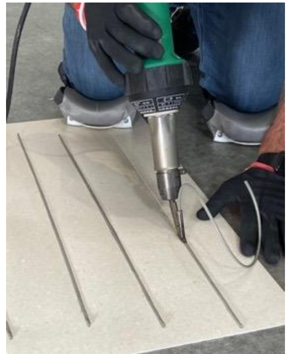
Figure 22 - Always perform practice welds.
