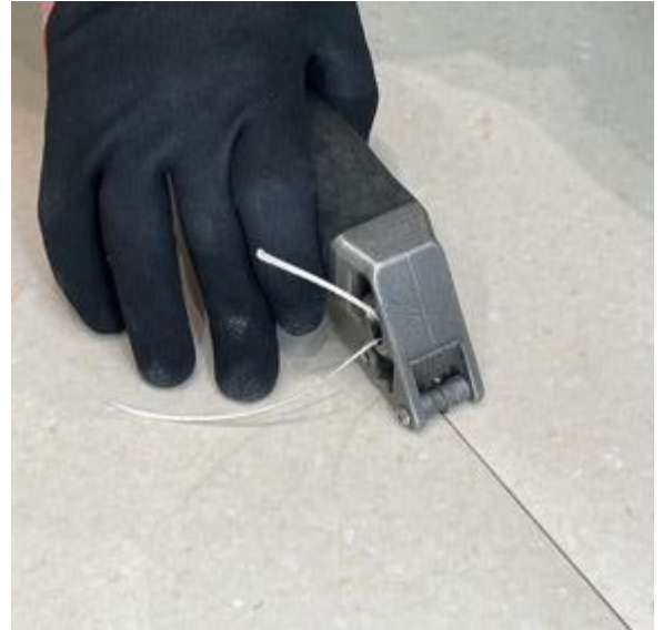
Figure 19 – Depicts the grooving of a seam using a push-type groover.
