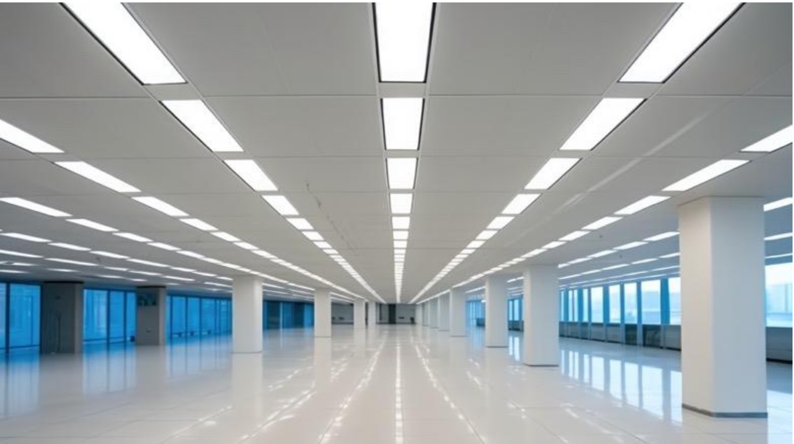
Figure 4 - Service lighting should be fully operational before installation begins.
