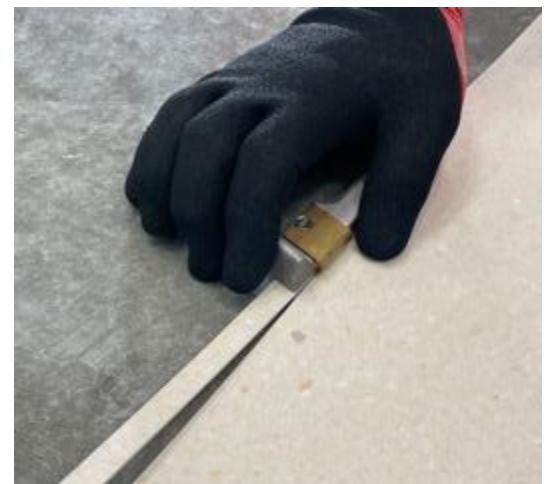
Figure 16 – Trim the factory selvage from the edge of the roll for proper seam construction.
