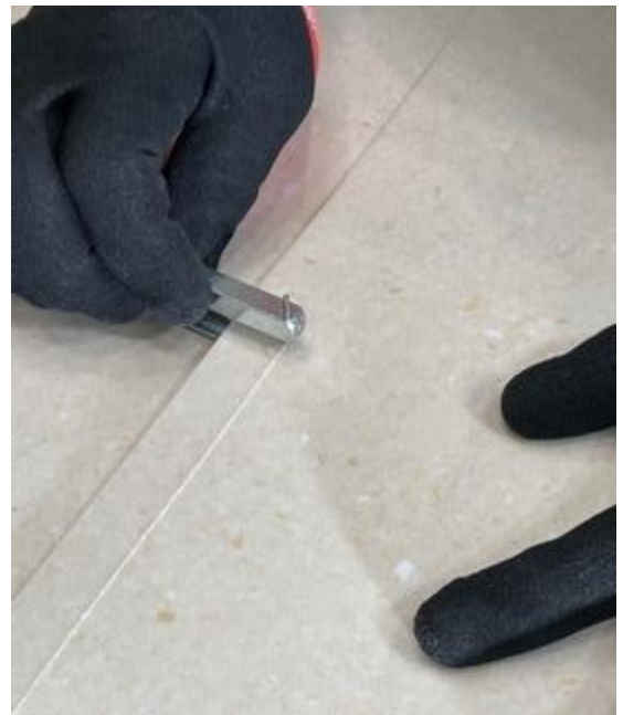
Figure 17 - Depicts the recess-scriber scoring the top sheet of flooring.
